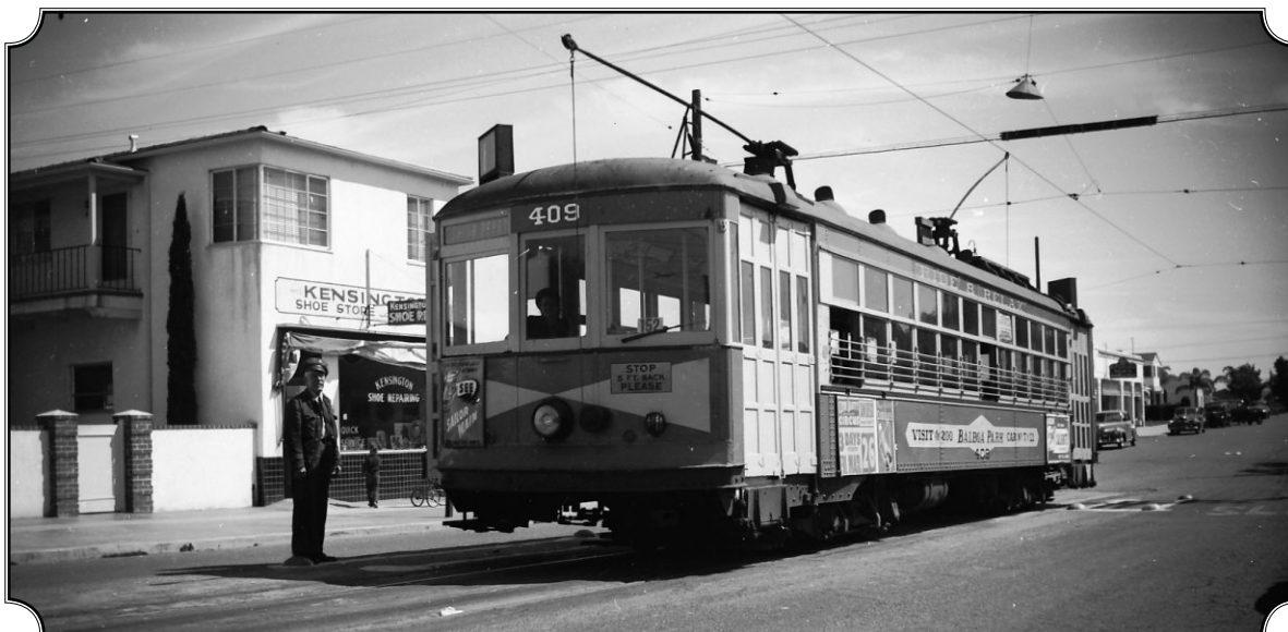
SDER 409 Line 11 Adams Ave. Terminal
